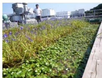
Roof-top greening with a thin-layer/fixed soil system (top) and a wetland type (bottom)
